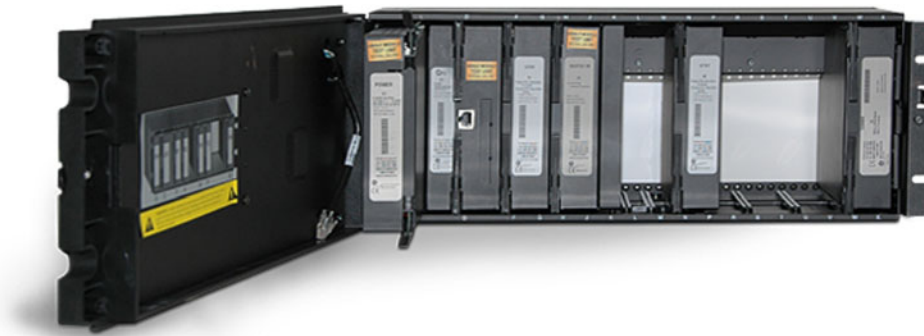
Figure 11-26: Modules inside relay with front cover open (enhanced front panel)
